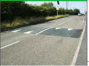
Tapered humps (humps that are not completely kerb-to-kerb) with a curved top surface. Minimum length 3.7 metres with a height of 65-100mm.
