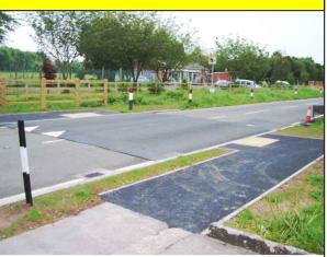
Normally full width of the road with a minimum 6 metre flat top to cater for easier movement of long vehicles.
